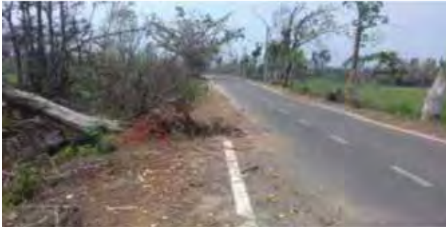
Tree uprooting and damages to berms
