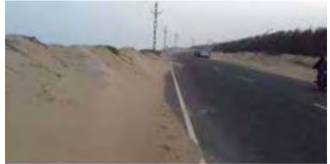
Sand accumulation on a coastal road
