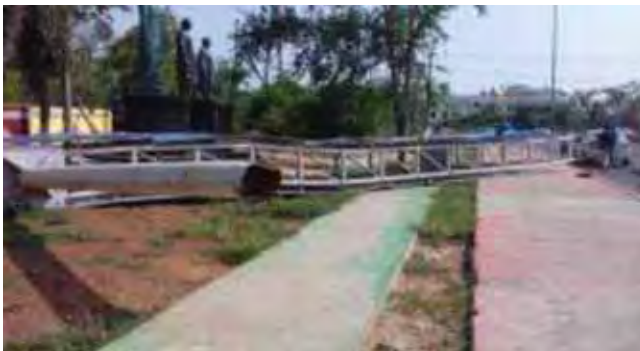
Road signs/gantry dislodging on urban roads
