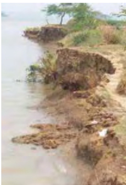
Location: Rajnagar Block, Kendrapara District – washed away portion of Keredaga Atlang Saline Embankment
