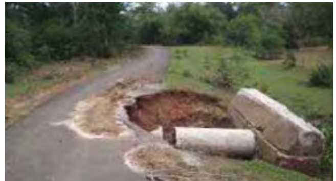
Culvert/embankment damages
