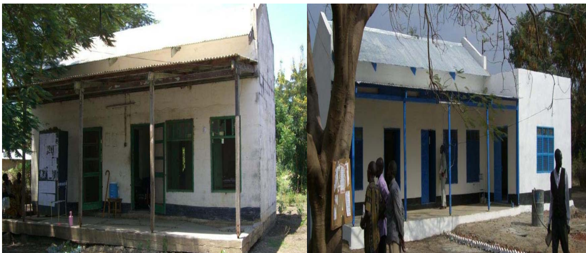
Malakal labour office before and after the renovation
