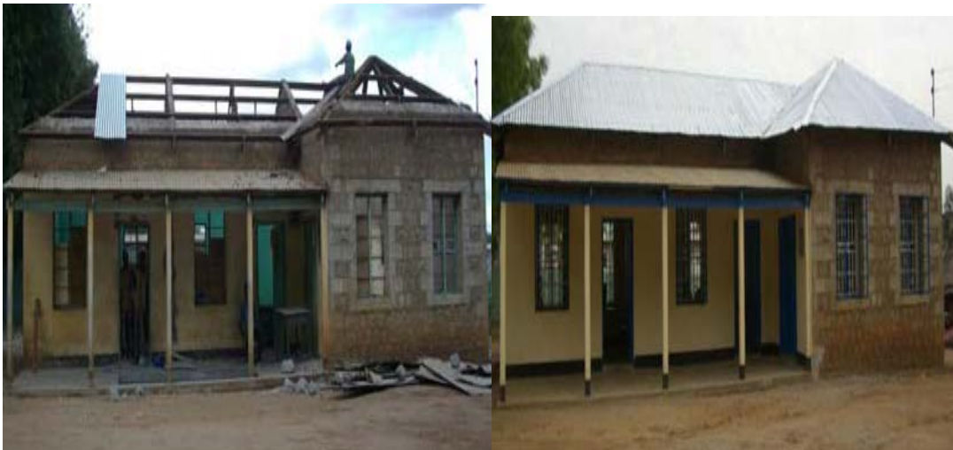
Juba labour office before and after the renovation
