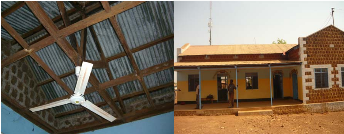
Wau labour office before and after renovation
