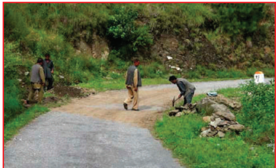
Figure 8: Workers performing routine maintenance
