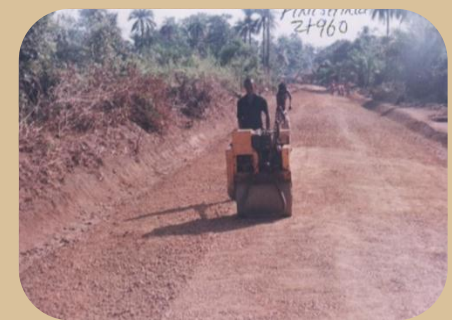
Compaction after spreading and watering
