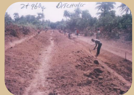
Ditching and preparing the road
