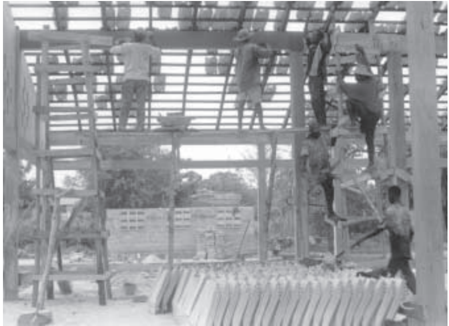
The markets were roofed using locally-made tiles. The walls were built with bricks made from clay extracted directly on the site.
