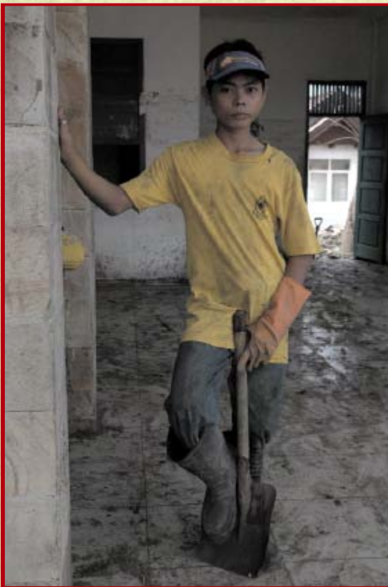
14 year-old Salatin works on this site in Banda Aceh for a Medan-based construction company. Children between the ages of 15 and 17 living in the camps for displaced persons in Aceh are the target of new training programmes launched by the ILO in March. In the coming months, the IPEC programme will be further extended, with a particular focus on vulnerable older children.
