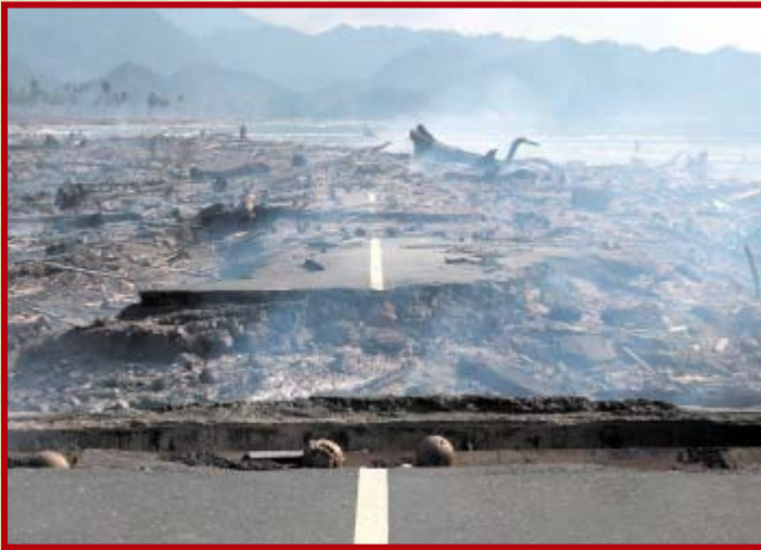
The road system has been badly damaged by the Tsunami. Rebuilding basic infrastructure will quickly generate jobs and income.
