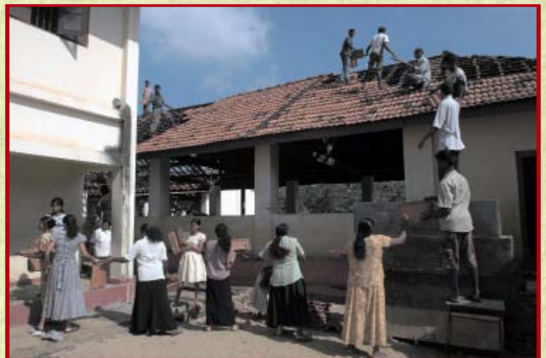
Ginthota, recovery of materials from the school before demolition.
