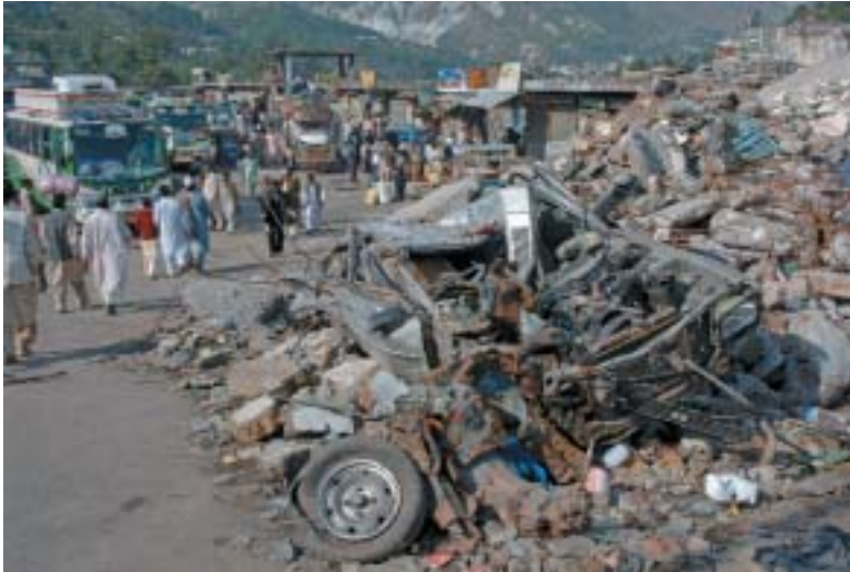
The remains of the bus station at Muzaffarabad, the city where the epicentre of the earthquake was located.
