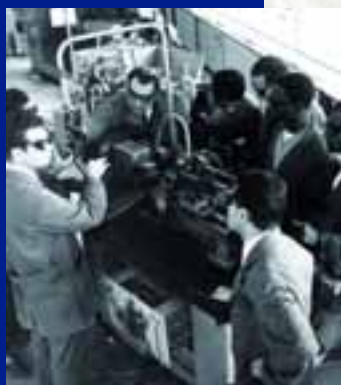
A Turin Centre training course, February 1969. A multilingual instructor explains the operation of a modern automatic lathe, run on an electro-pneumatic system, of the type used in making components for the automobile industry
