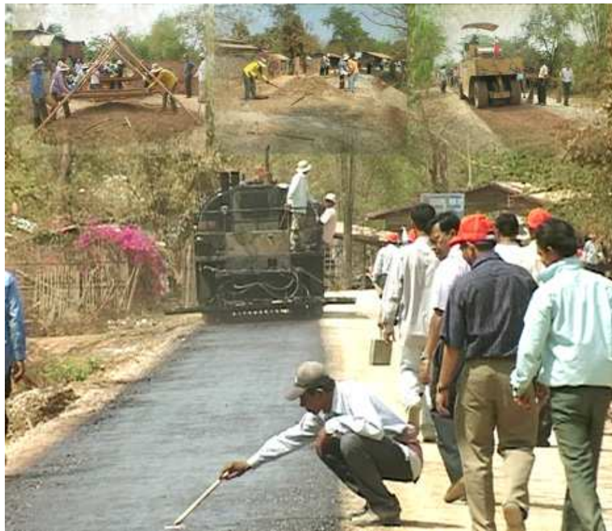
Construction of Trial Sections – ADB/JFPR Project TA-9048
