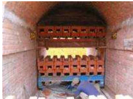
Figure 21. Fireman arranging bricks in the eco-kiln
