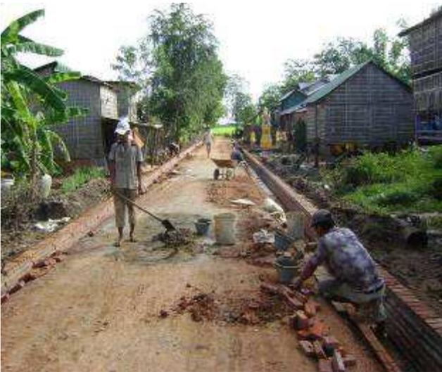
Side drains with brick masonry lining
