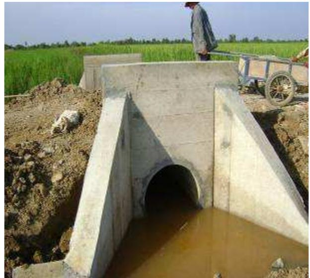
Completed culvert with abutments
