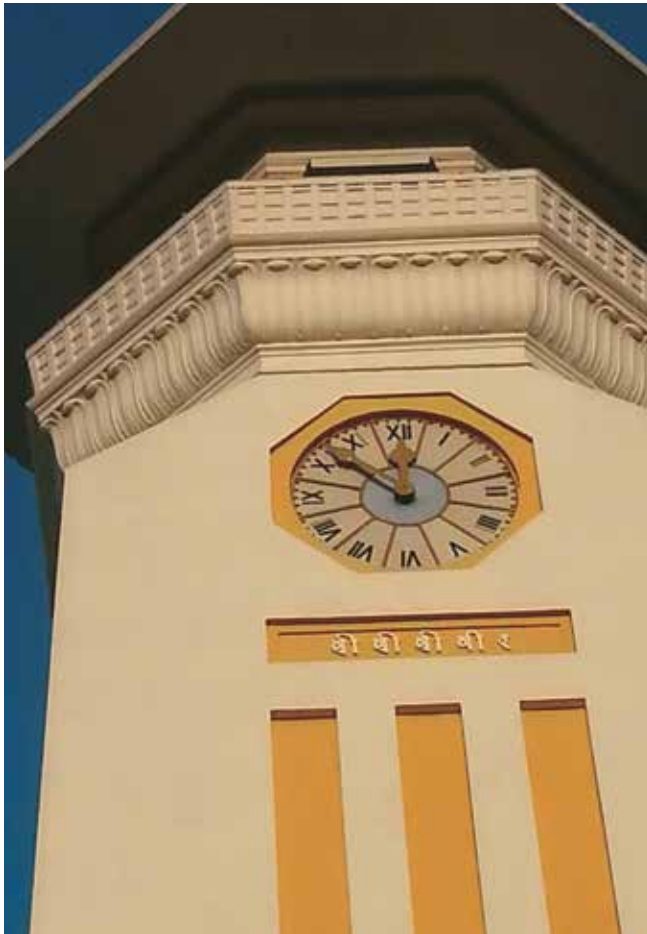
Time stood still at 11:56 local time on 25 April, 2015 when the earthquake struck in Nepal (GhantaGhar, the public tower clock in Kathmandu). © ILO Nepal/S. Gurung
