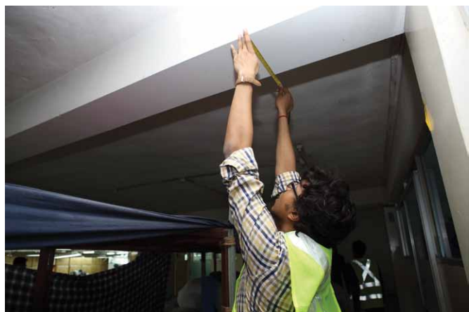
Following safety inspections, remediation work is now top priority in the RMG sector
