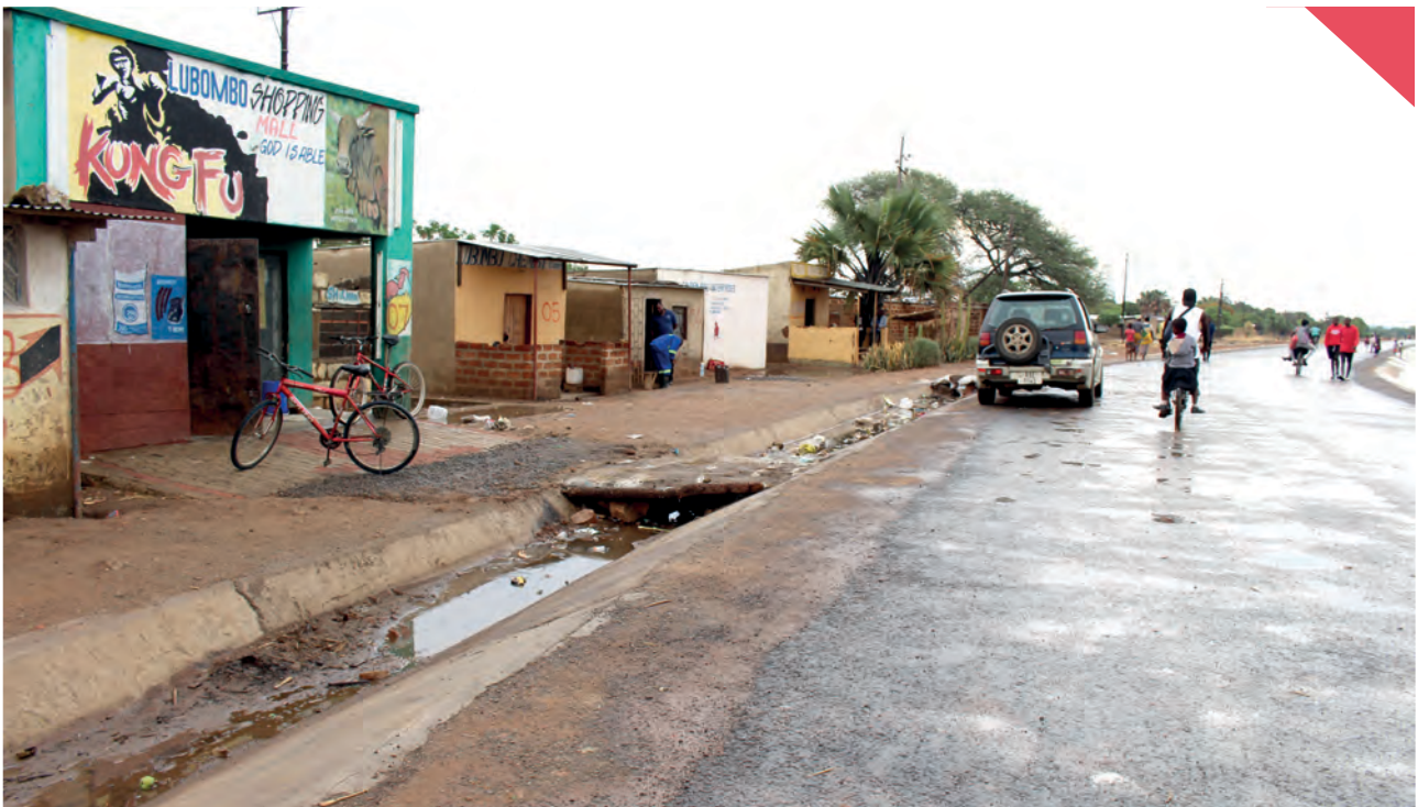
Part of the road constructed using labour-based technologies
