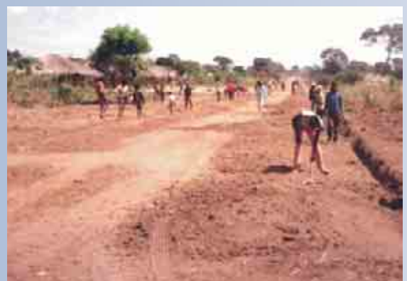
Drain and road excavation
