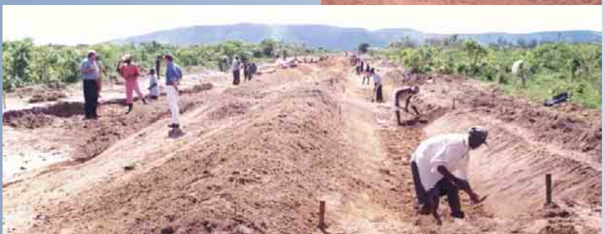
Drain and road excavation
