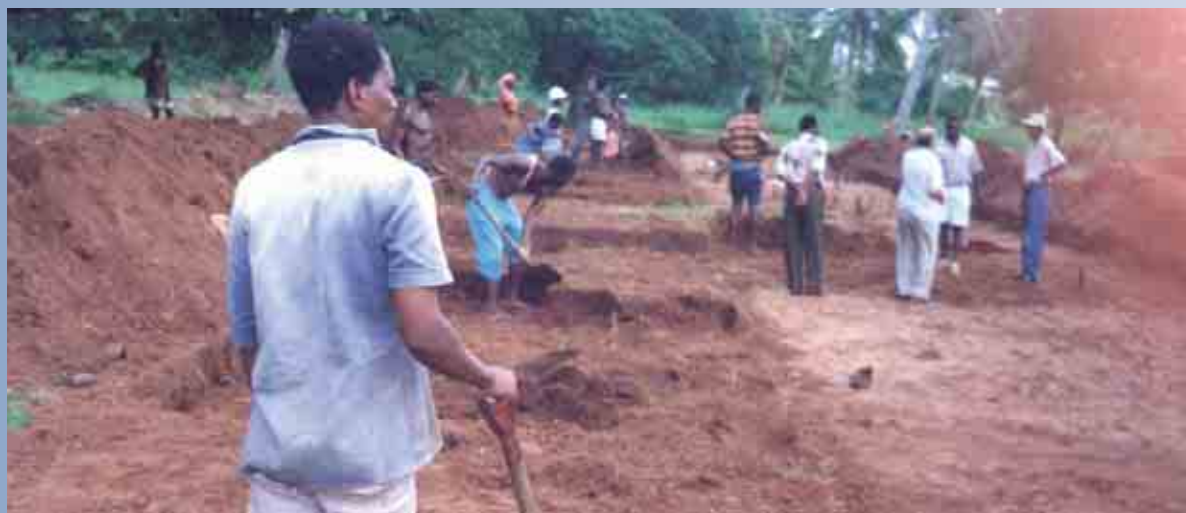
Removal of top soil
