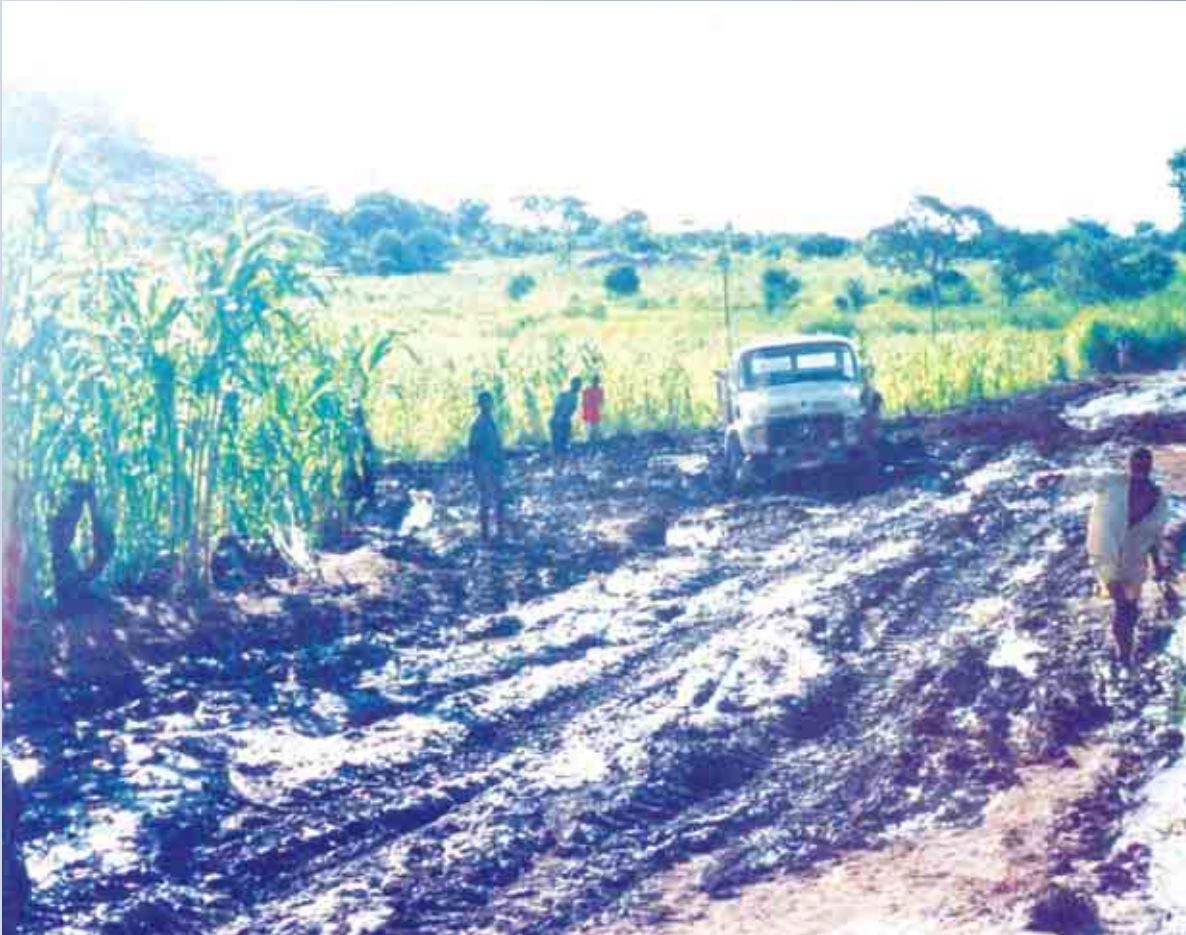
Bad road during rainy season
