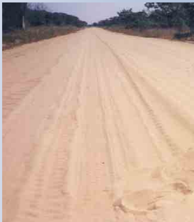
Trials with soil stabilisation
