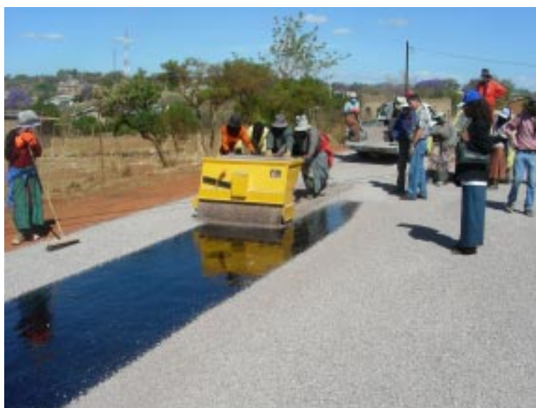
Spreading stone chips using a manual spreader
