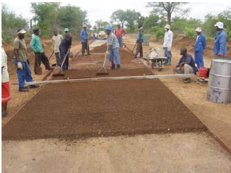
Preparing the sub-base at Gundo Lashu
