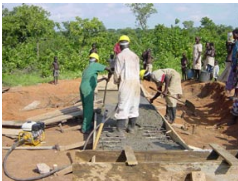
Damanko-Pibilla road Nkwanta District A4 contractor preparing a culvert deck
