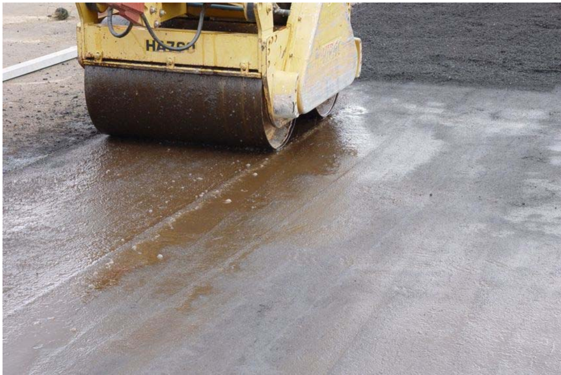
Figure 12: Compaction until surface is saturated with brown liquid
