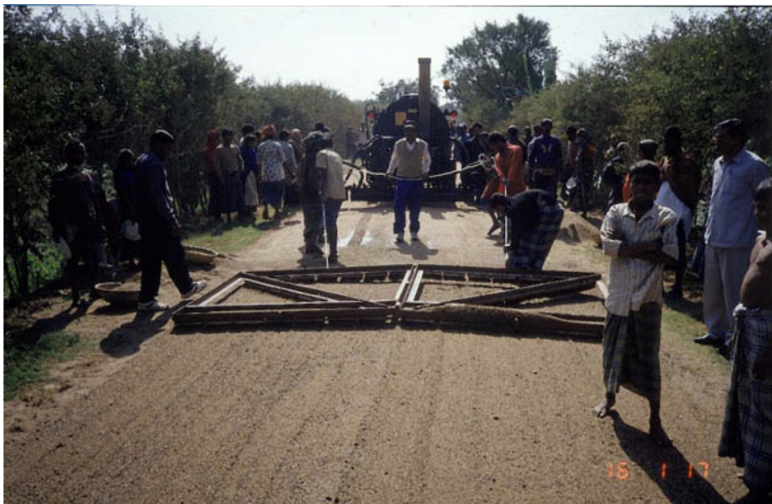
Figure 3: Levelling of aggregate for Otta Seal using a drag broom
