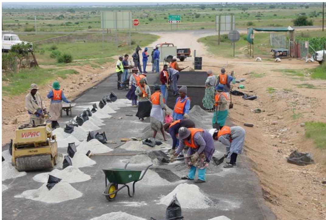
Figure 10: LBS Asphalt being mixed on site
