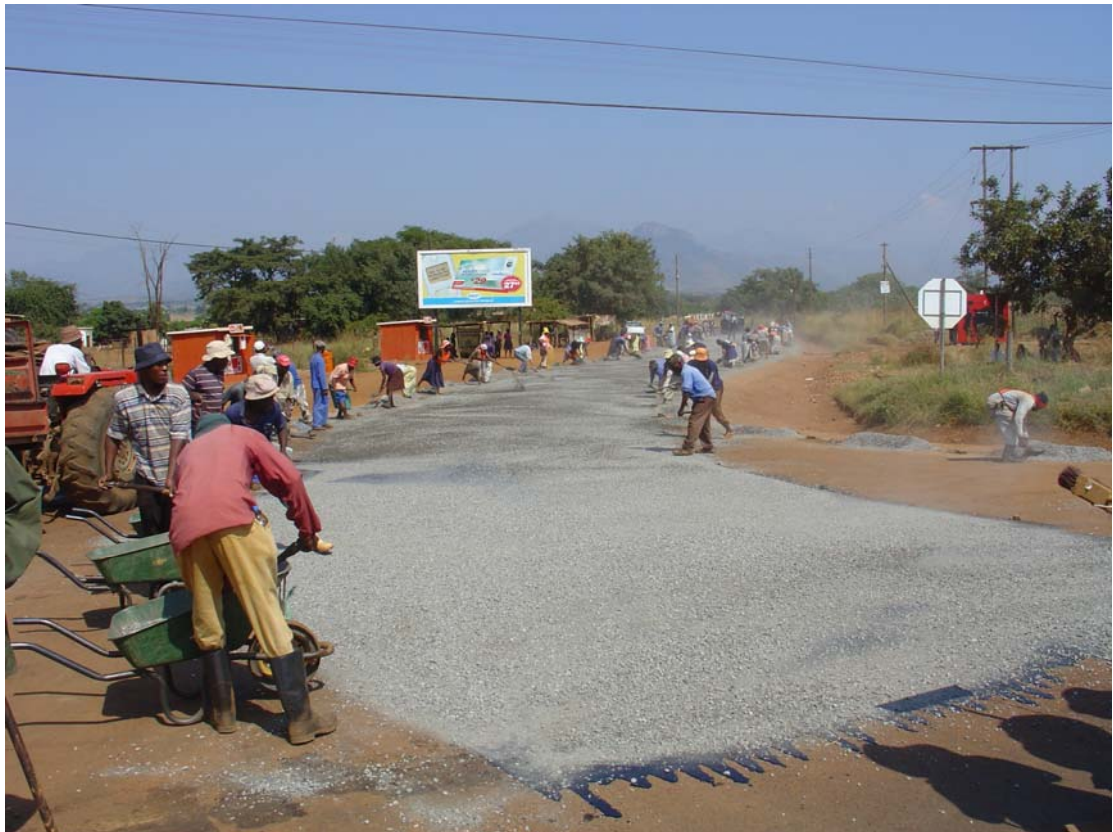
Figure 5: Hand spreading of aggregates for Otta- or Grav Seal
