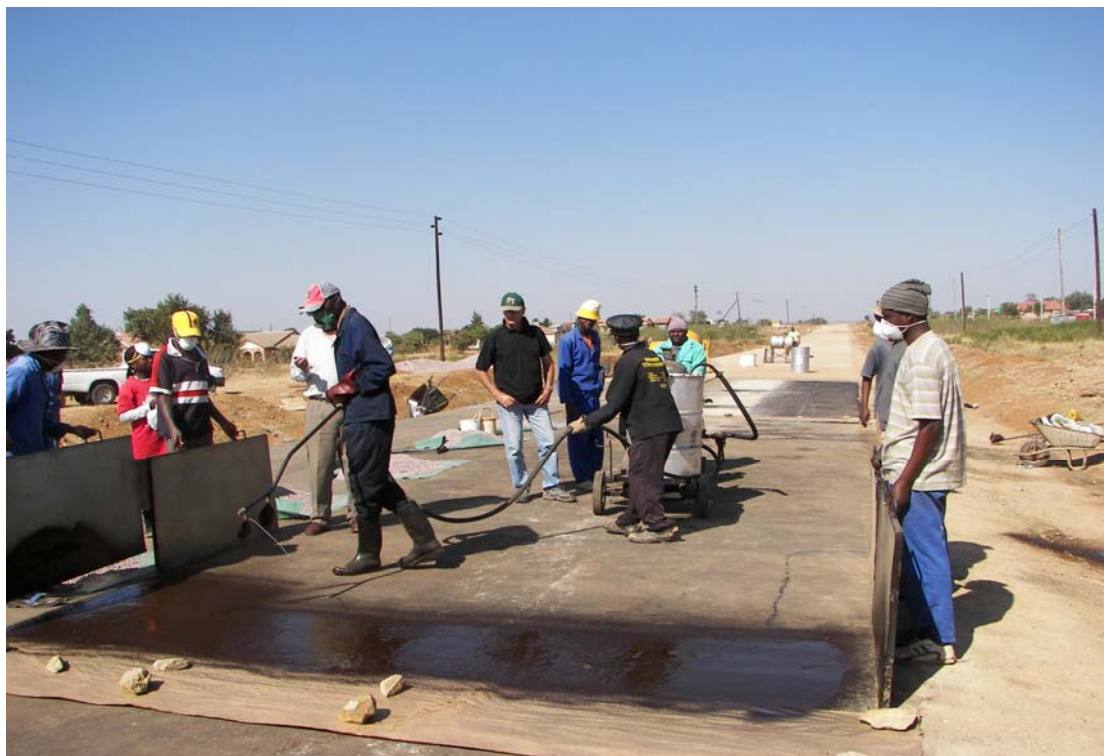
Figure 11: Spraying of tack coat with a motorised hand sprayer
