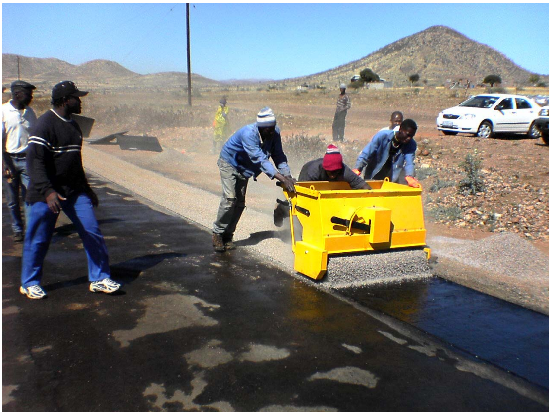
Figure 9: The "chippie" greatly simplifies the uniform spreading of aggregates.
