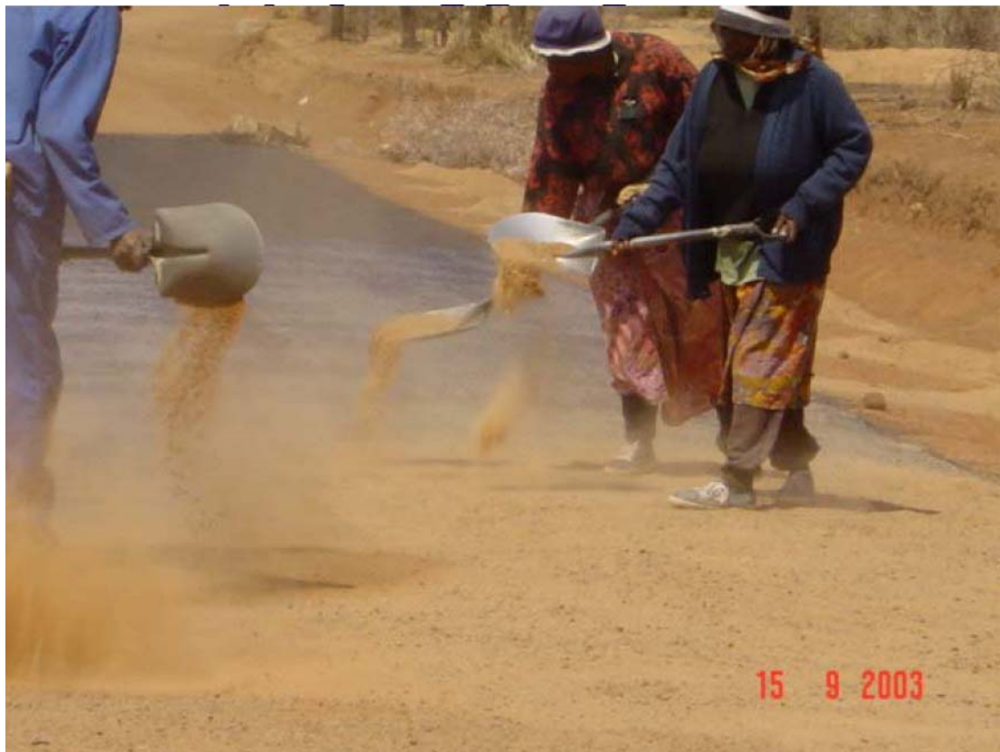
Figure12: Spreading of sand for a Sand Seal. A flipping of the shovel will make dust fly away with the wind. The sand should be broomed to an even layer before rolling.
