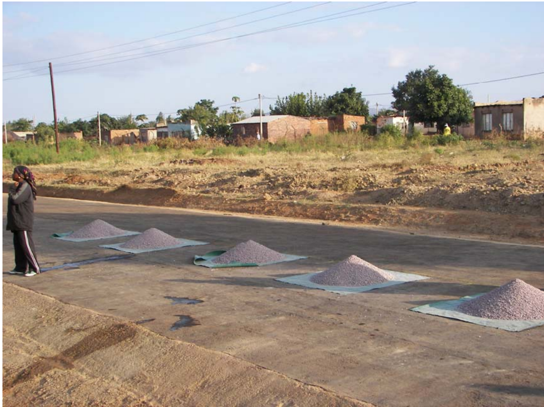
Figure 7: Spotting of aggregates in accurate quantities for the area to be covered. The amount is measured in a half drum open on both ends placed on the plastic sheet and lifted off once the required quantity has been filled in the drum.
