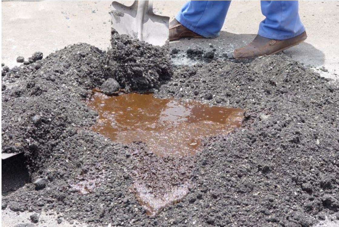
Figure 11: Emulsion is added to the dry mix of filler and aggregates and mixed by hand
